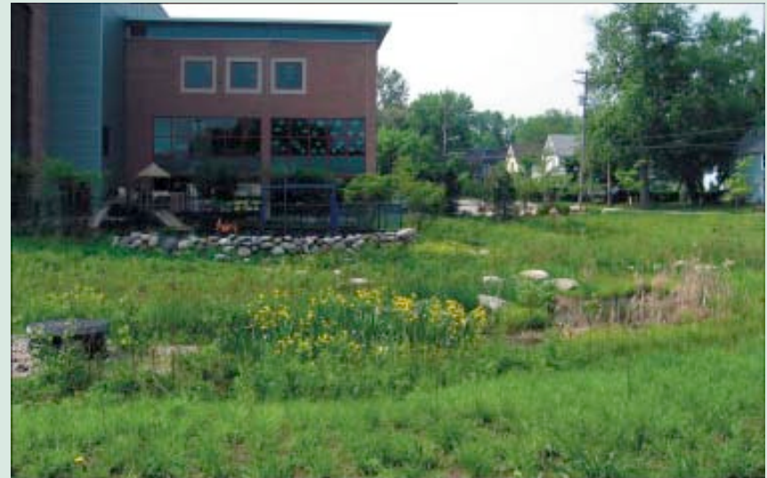
Stormwater retention retains water on site AND serves as an amenity
