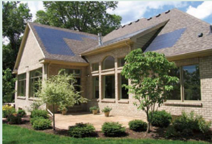
BIPV with varied orientation (Ohio)
